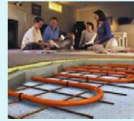
Radiant Floor Heating
